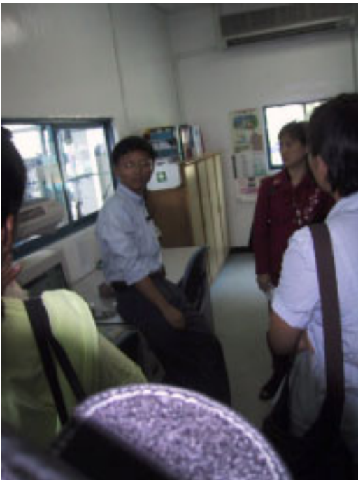
Our host, Mr Ong, telling us more about control room operations.
